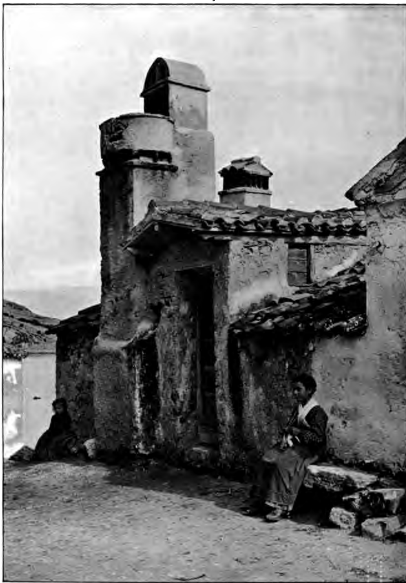
CHIMNEYS AT BESCA NOVA
